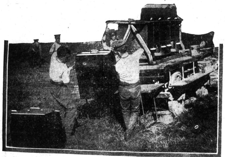
The new field kitchen, filled with removable ovens, by means of which one hundred meals of soups, joints, vegetables, tea, etc., can be served immediately when a halt is called. Very little coal is required, the fire being kept going with wood or dry refuse found on the field. A rack over the stove provides facilities for drying clothes.
