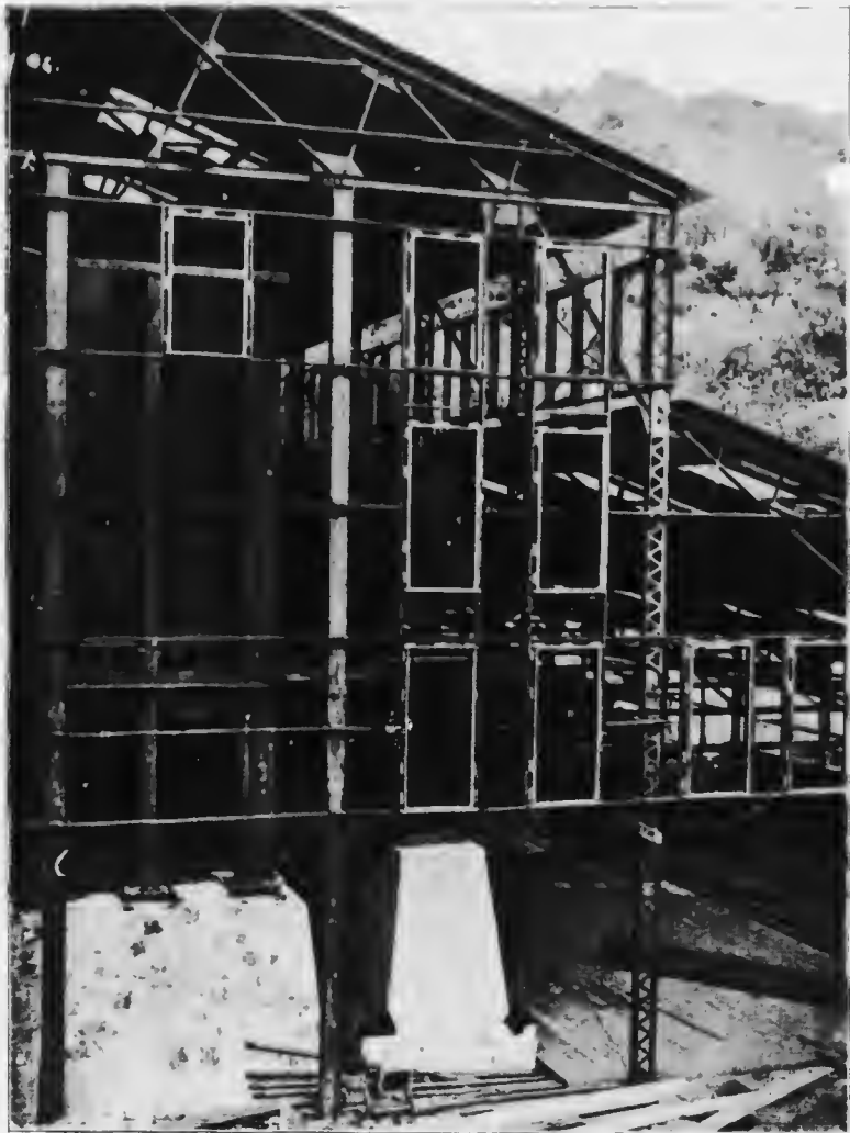
Fig. 45 Bustos Mill, in Course of Construction.
