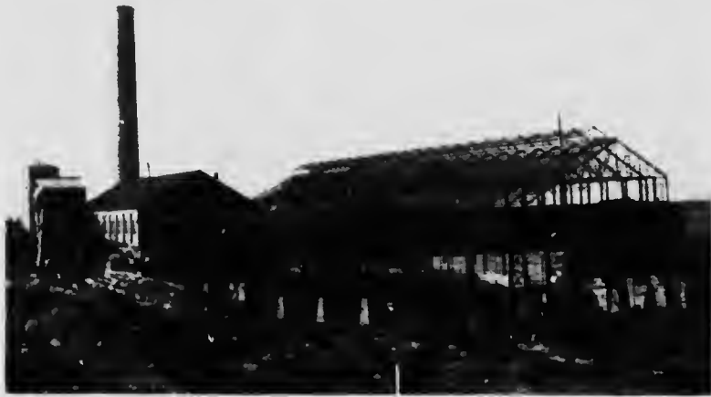
CONISTON SMELTER IN COURSE OF ERECTION, OCTOBER, 1912
