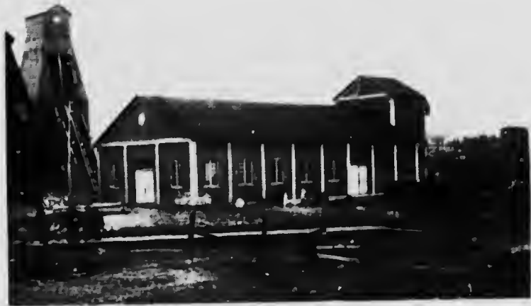
WORTHINGTON MINE (POWER HOUSE) Coal and Electric Railway in the foreground
