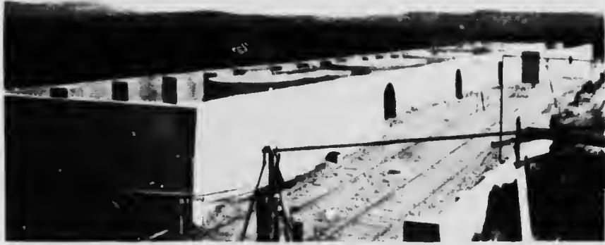
A PART OF THE FOUNDATIONS OF CONISTON SMELTER JAN. 1912
