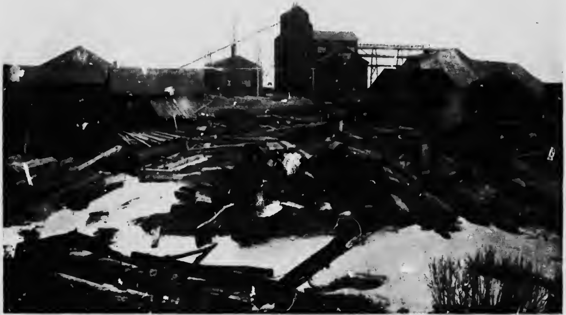
VICTORIA MINE General View of Plant
