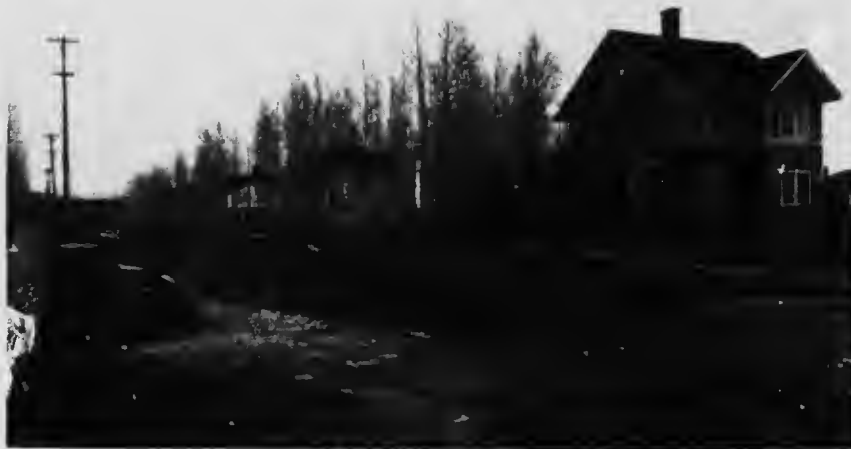
CONISTON PLANT Looking north along First Avenue, Coniston Village
