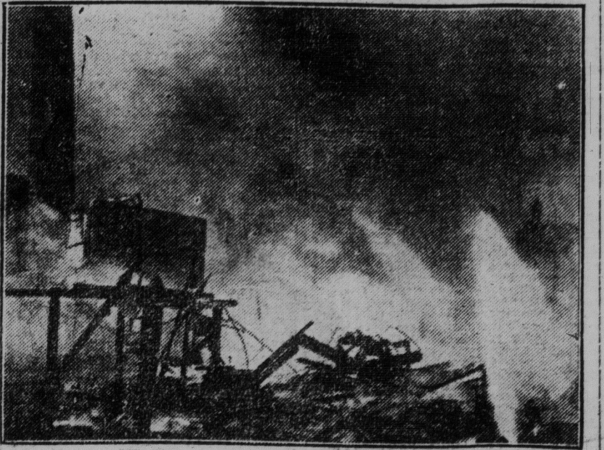
Fighting the fire from the rear, as seen from the top of a building behind Balmuto street.
