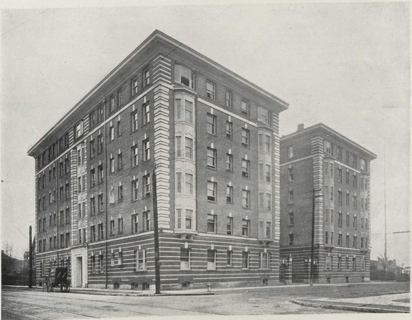
Holly Lodge, Largest Apartment Block in Vancouver, B.C. Wright, Rushforth & Cahill, Architects; Barr & Anderson, Plumbers; Dalton Bros., Contractors. Equipped with Standard Ideal Plumbing Fixtures.
