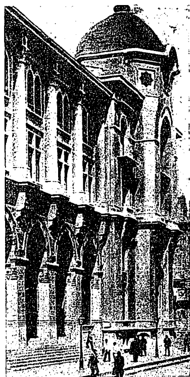
ENTRANCE TO POST OFFICE.
