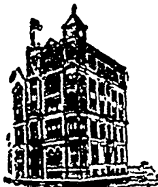
HEAD OFFICE BUILDING, MONTREAL.
