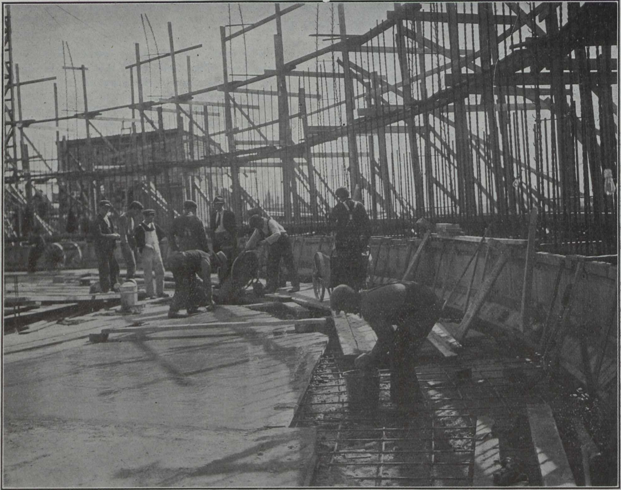
Floor Construction Showing Reinforcement.
