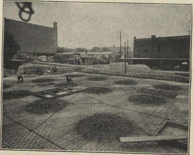
Mushroom Frames and Rod Reinforcement Running Over Them.
