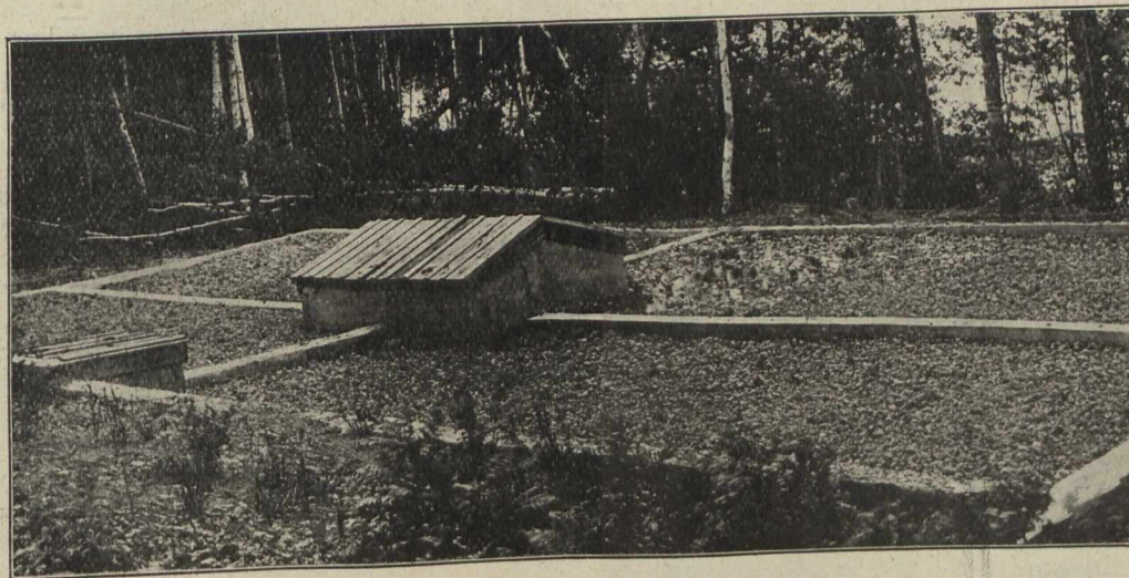
Contact Beds of Large Plant Built in Concrete.
