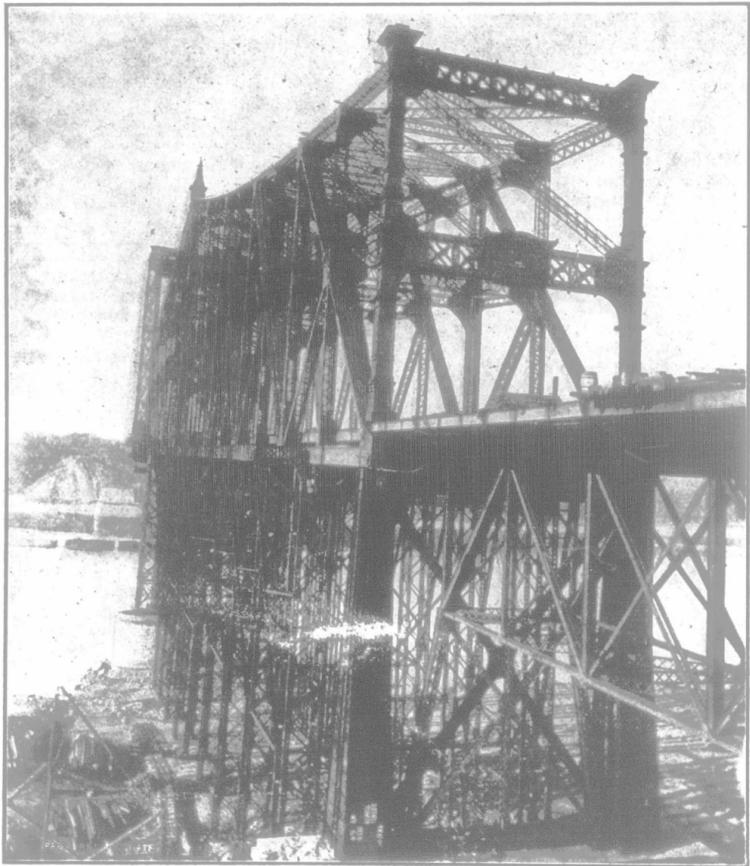
QUEBEC BRIDGE, SHOWING THE "FALSEWORK" OR SCAFFOLDING, AND UPPER BRACES OF 20 THICKNESSES OF STEEL.
