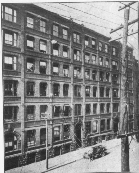
WESLEY BUILDINGS—AS THEY ARE NOW. TEMPERANCE STREET FRONT.
