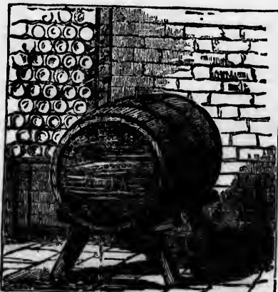
A LEAKING TAP IS A GREAT WASTER.
