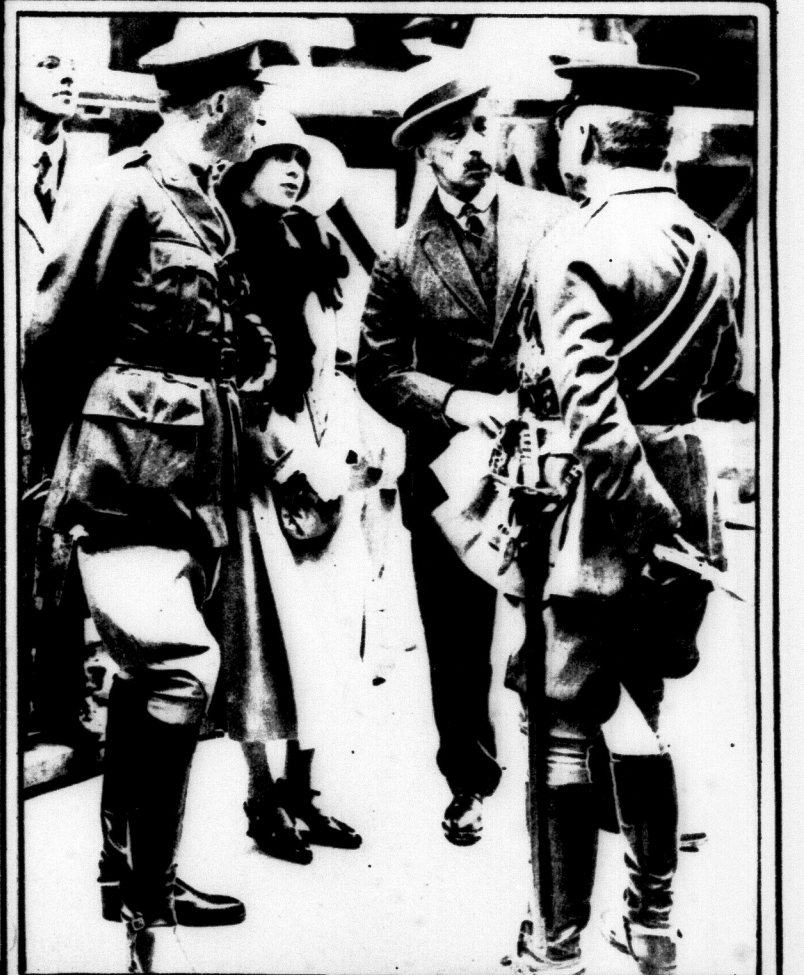
Viscount Lascelles and Princess Mary inspect the partly-finished Scottish war memorial at Edinburgh
