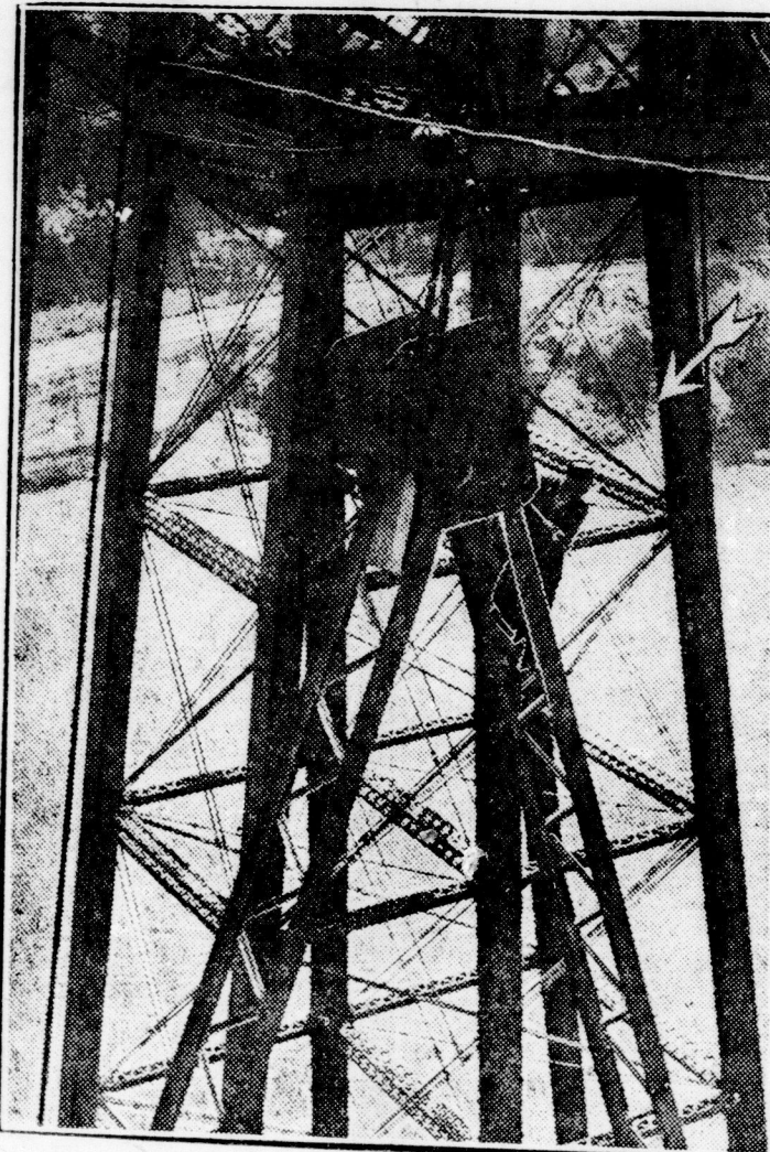
An iron worker photographed a hundred feet above the Niagara River while working on the Canadian end of the Michigan Central bridge now in the course of erection
