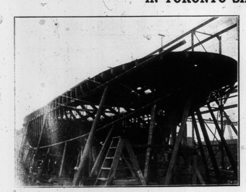
Framework of a new steel tug, now under construction at the Toronto shipyards, and which will ready for launching early in May.
