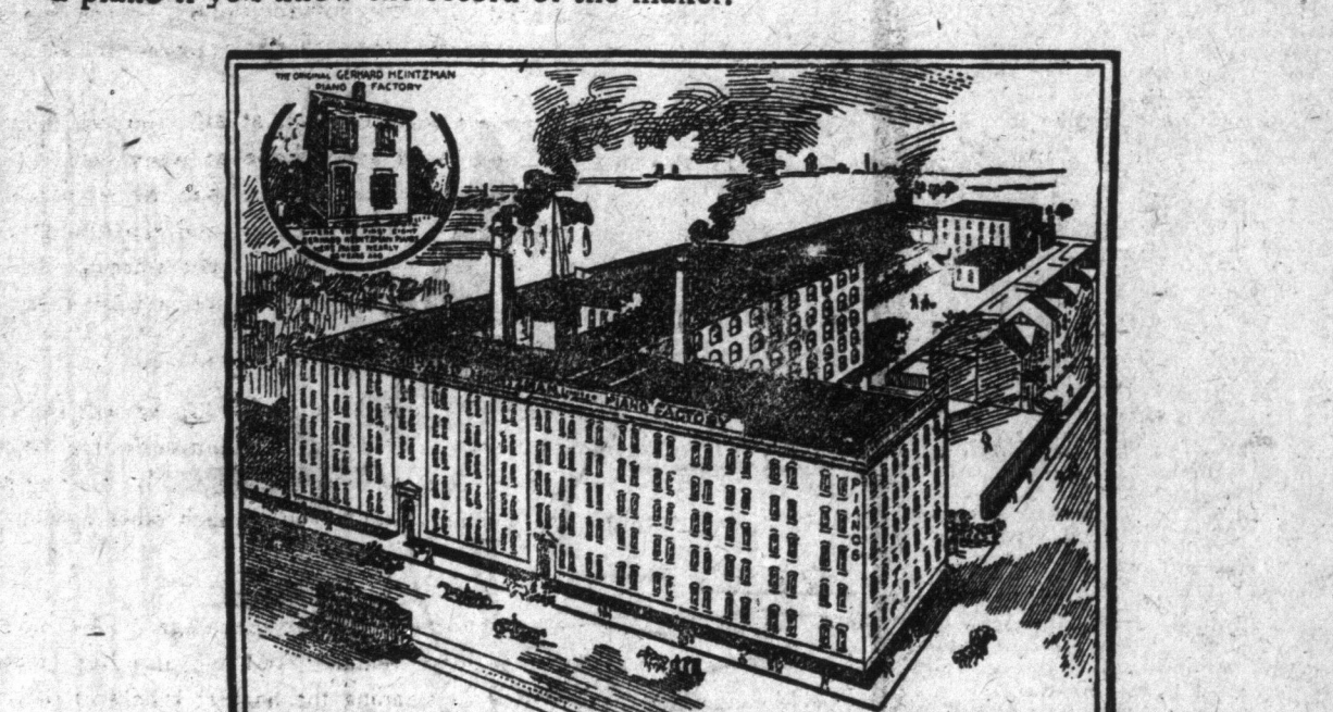
Bird's eye view showing the enormous plant of Gerhard Heintzman, Limited, grown to these proportions through the merits of their pianos.
