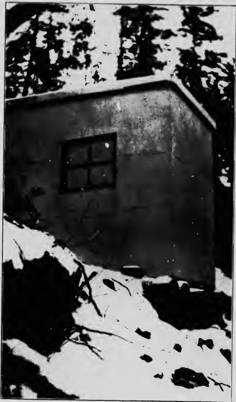
Adams River Automatic Gauge House.
