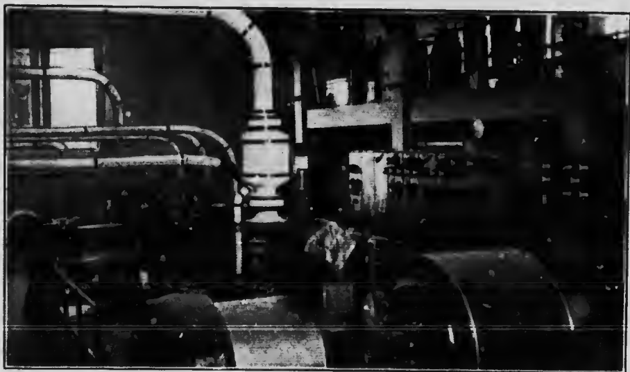
Interior Sub-Station, City of Kamloops.
