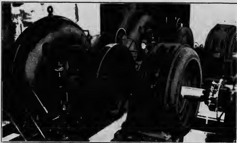
Interior Barriere River Hydro-Electric Power House, Municipal plant for City of Kamloops. Photograph by courtesy of Messrs. Ducane, Dutcher & Co., Consulting Engineers, Vancouver.
