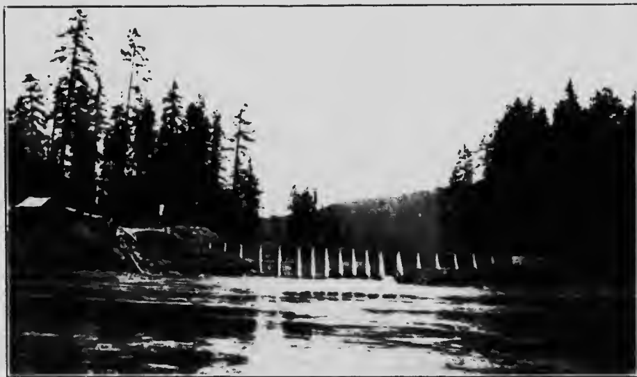
Impounding dam of Puntledge River Hydro-Electric Installation on Puntledge river near outlet from Comox lake.
