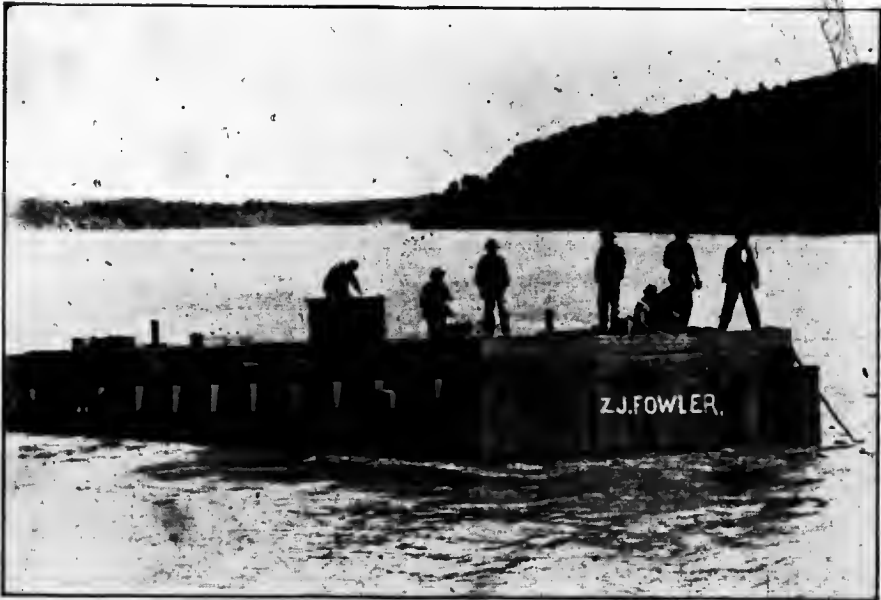
Photo 2.—Showing Caisson on way down from shipyard to Bridge site.
