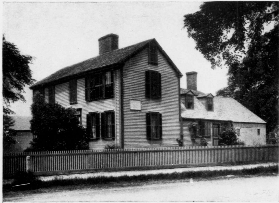
THE HANCOCK-CLARKE HOUSE
