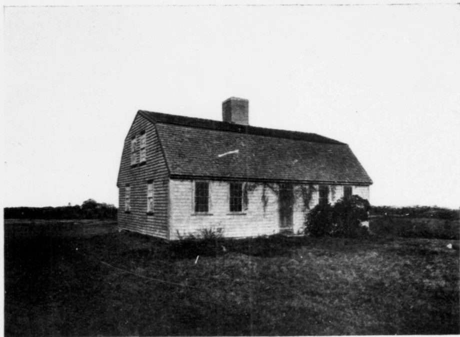
THE STANDISH HOUSE, DUXBURY
