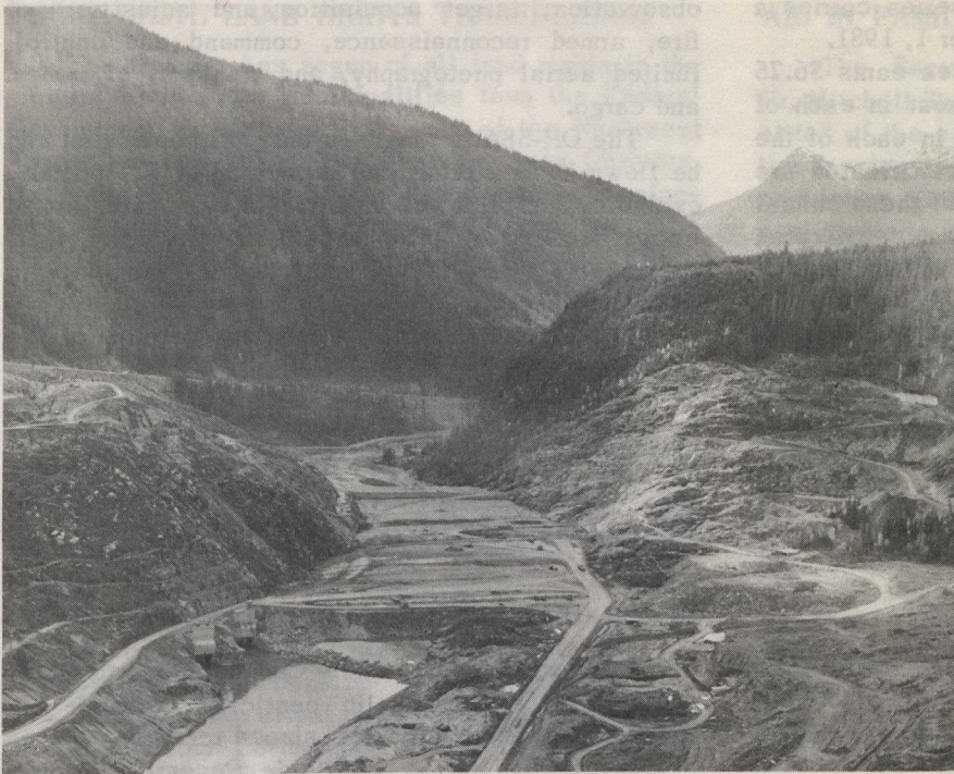
The aerial photo of the Mica damsite, near Revelstoke, B.C., looking downstream, shows intakes for the diversion tunnels (near bottom left of picture).
