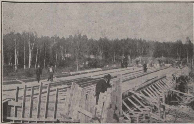
Cumberland Street Bridges; View of Form Work in Place.
