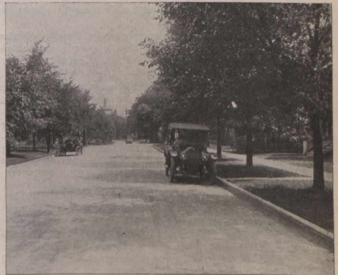
Finished Dolarway Pavement.
