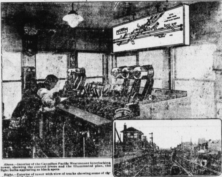
Above.—Interior of the Canadian Pacific Westmount interlocking tower, showing the control levers and the illuminated plan, the light bulbs appearing as black spots. Right.—Exterior of tower with view of tracks showing some of the signals switch plant.
