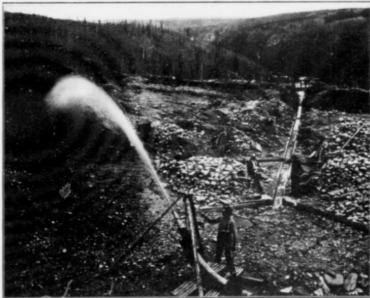
Hydraulic mining frozen material on a small scale on Gold Creek, a tributary of Flat Creek, Yukon.
