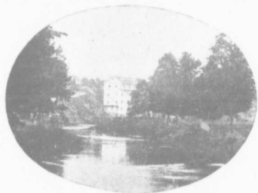
VIEW FROM REAR OF FLOUR MILL
