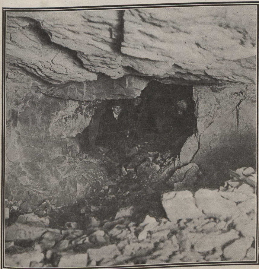
On December 10, as Promised, Engineer Brown's Men Blasted the Last Few Feet Between the Two Headings and Completed the C.N.R. Tunnel Through Mount Royal. This Picture Shows the Final and the First Men Through.
