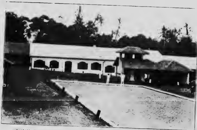
STONE FLOOR FOR DRYING CACAO-BEANS IN THE OPEN AIR
