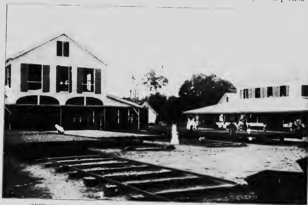
SURINAM. DRYING COFFEE ON PLATFORMS WHICH CAN BE RUN UNDER SHELTER
