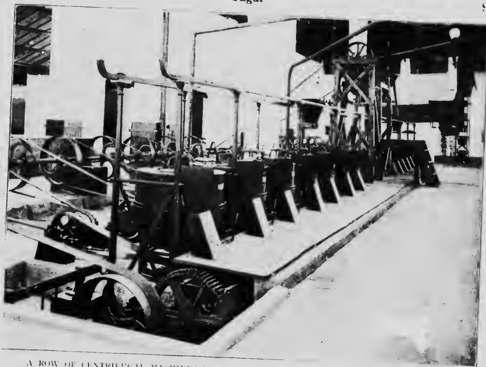
A ROW OF CENTRIFUGAL MACHINES FOR SEPARATING SUGAR CRYSTALS FROM MOLASSES
