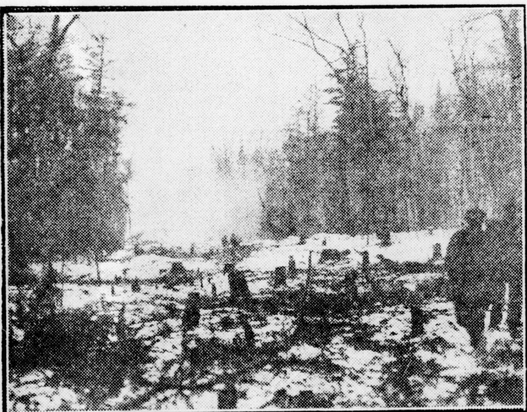
In 1927 motorists will be able to travel from Toronto to Cobalt, when the new gravel highway, from North Bay on, will have been completed. Here is shown a 66-foot cutting being made which will extend through sixty miles of bush
