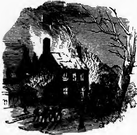
HOUSE ON FIRE.
