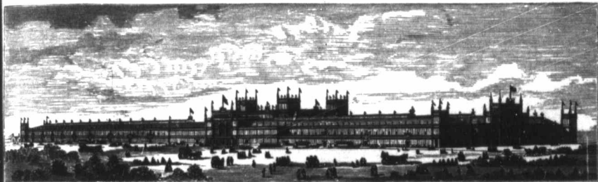
Main Exhibition Building.
