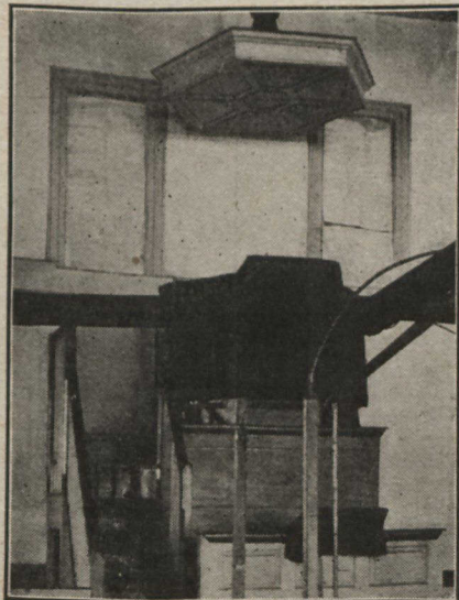
The pulpit of an old-time church; note the sounding board hanging from the ceiling.
