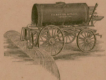
AUSTIN STEEL STREET SPRINKLER
