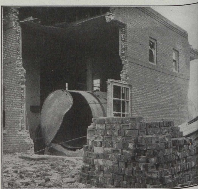
Results of Explosion of Water Storage Tank at Canora, Saskatchewan.
