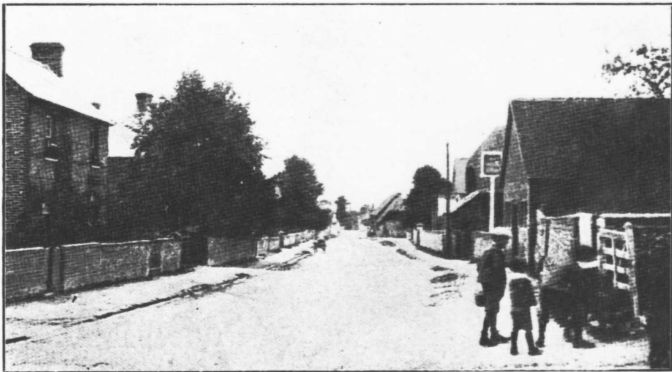
HIGH STREET, CHINNOR—LOOKING TOWARDS OXFORD.
