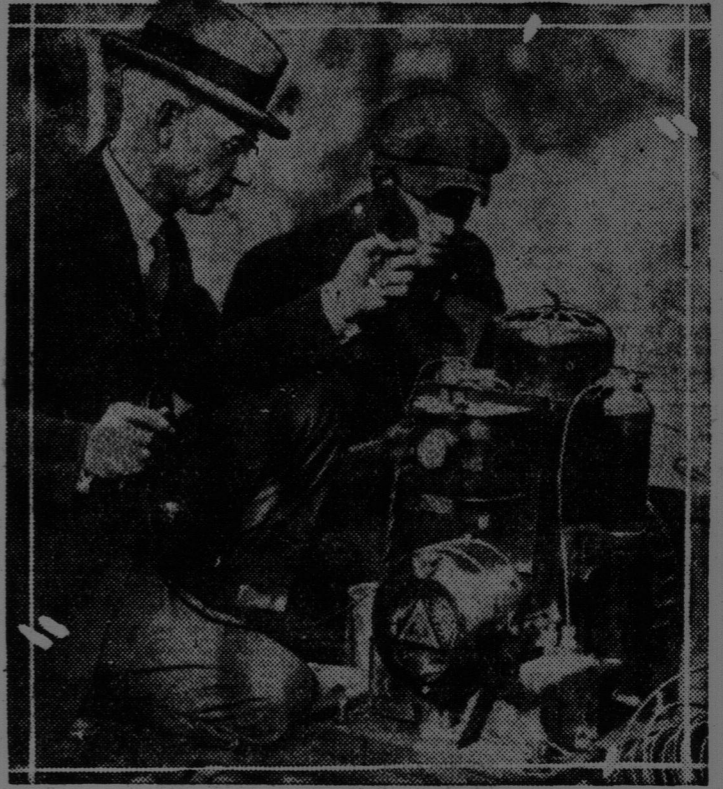
Upper picture shows where shaft was sunk to cave "tomb" of Floyd Collins at Sand Cave, Kentucky. Lower picture shows electrical plant at mouth of cave, which gave warmth to Collins over a light circuit. Over this circuit radio tests were taken to determine whether Collins was living.
