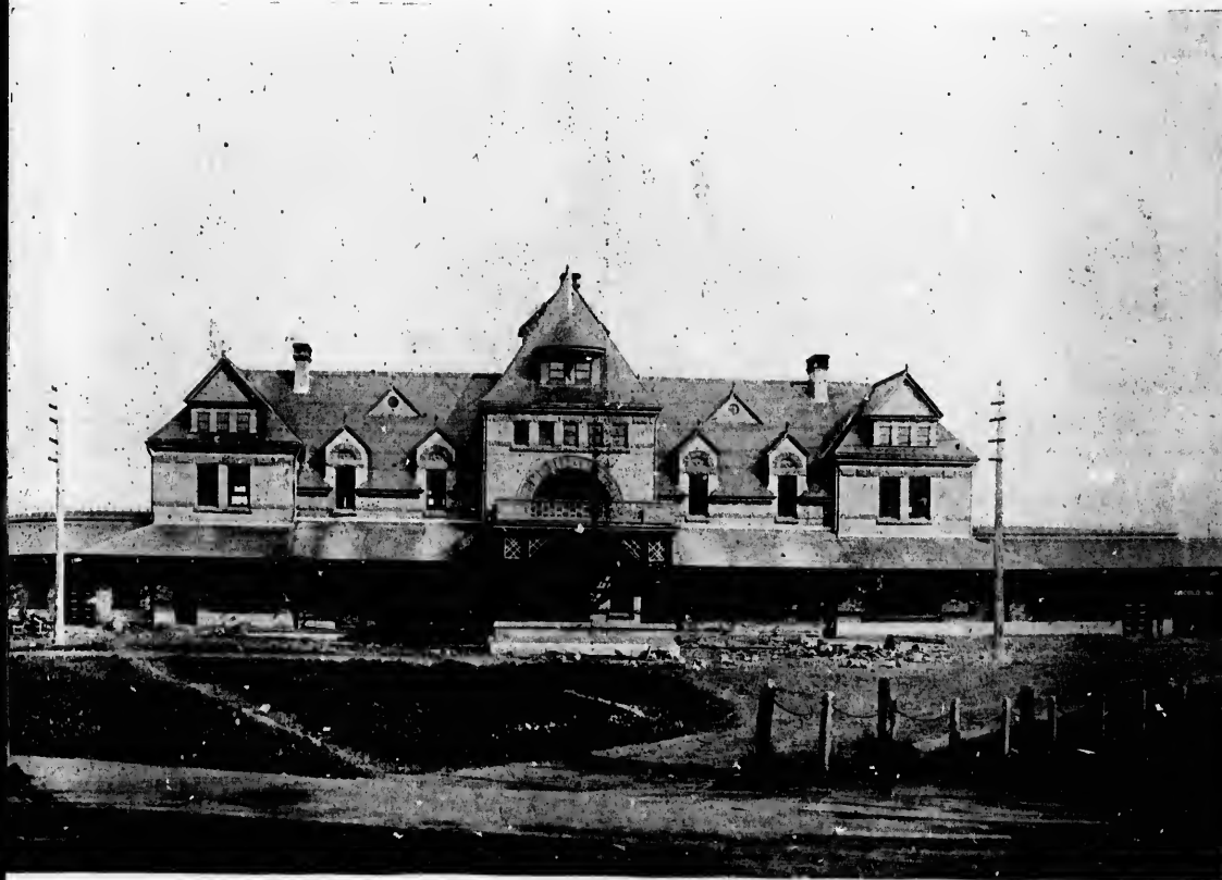
NEW INTERCOLONIAL RAILWAY STATION, MONCTON, N. B.
