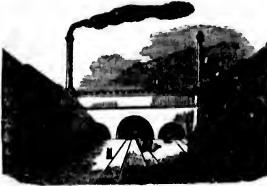
Entrance to the Railway Tunnel, Liverpool.
