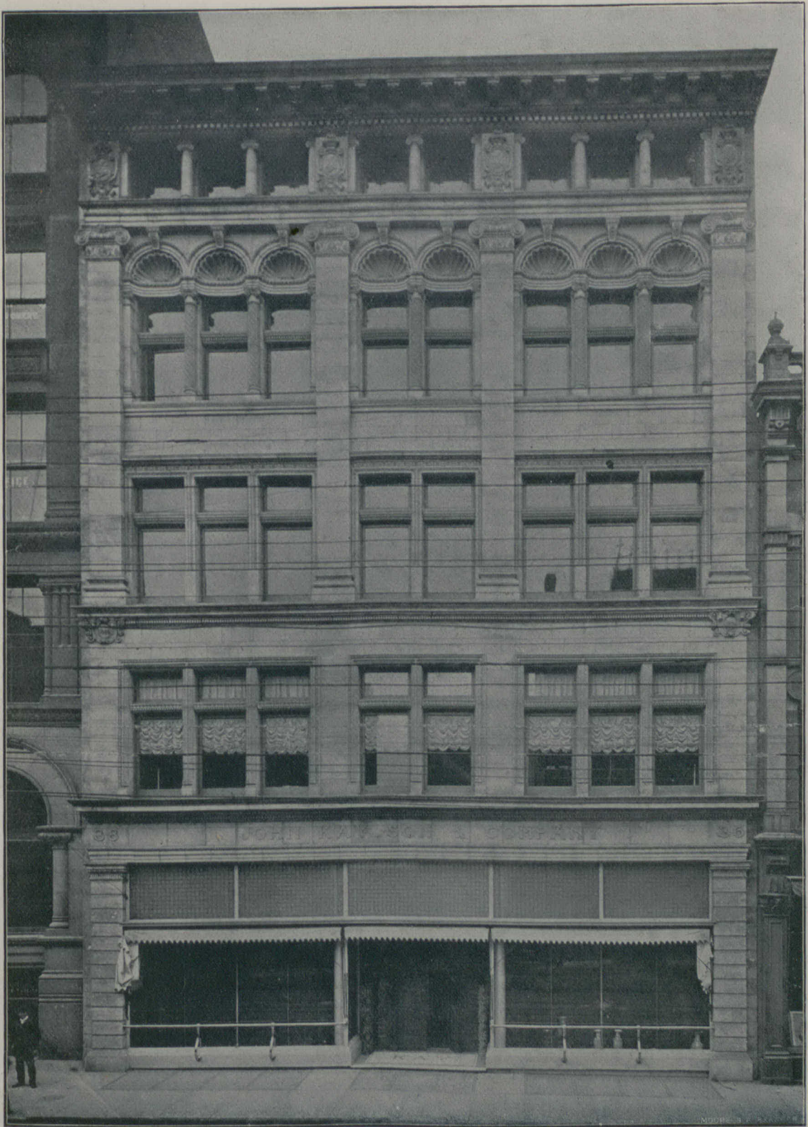
BUSINESS PREMISES ON KING STREET WEST, TORONTO, FOR MESSRS. JOHN KAY, SON & COMPANY. S. G. CURRY, ARCHITECT.
