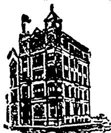
HEAD OFFICE BUILDING, MONTREAL.
