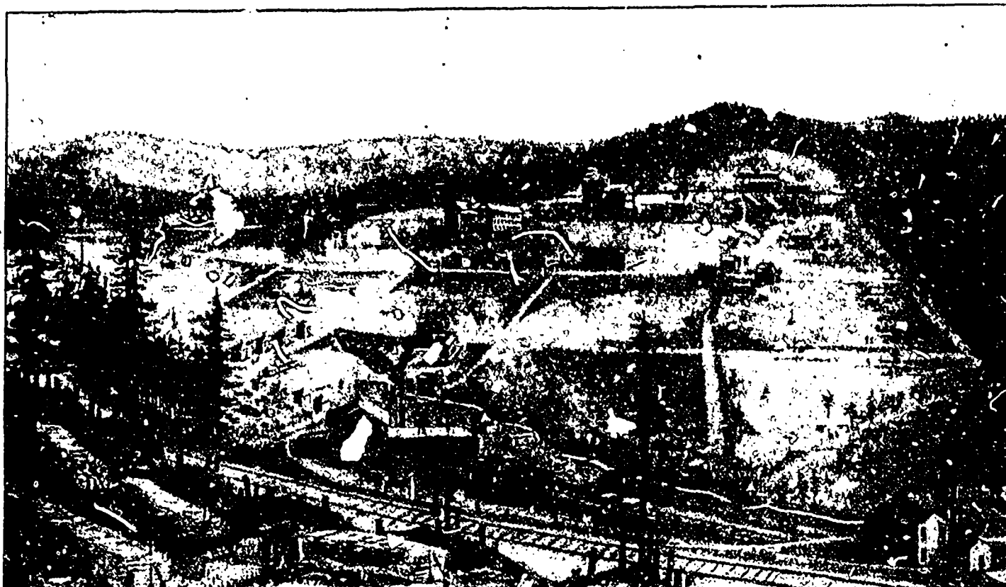
VIEW OF KNOB HILL MOUNTAIN SHOWING KNOB HILL, OLD IRONSIDES AND GRANBY MINES AND BUILDINGS AT PHOENIX.
