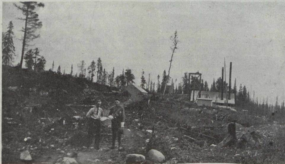
Matachewan Gold Mine, N. Ont.
