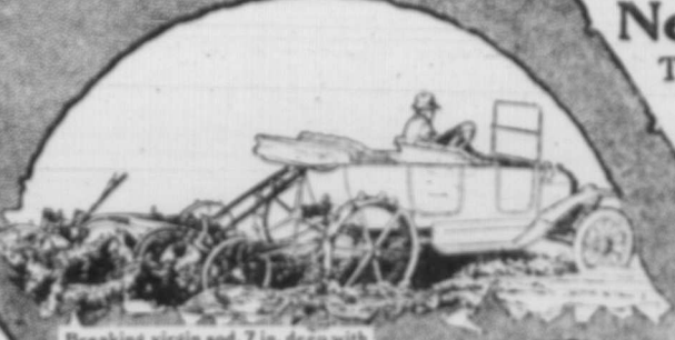
Breaking virgin soil, 7 in. deep with 2 bottom, 28 in. gang. (Reproduction from moving picture film.)
