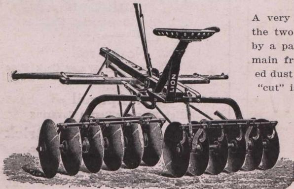
A very popular type. Staunchly built, the two disc sections are held in place by a particularly strong and rigid steel main frame, and run on highly polished dust proof bearings. The angle of the "cut" is controlled by one handy lever.
