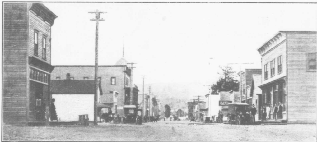
ONE OF MERRITT'S BUSY STREETS Photo taken May, 1911
