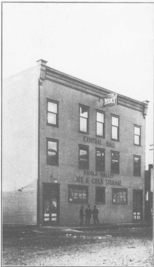
MERRIT'S COLD STORAGE BUILDING One of the largest and most up-to-date in the Interior of B. C.
