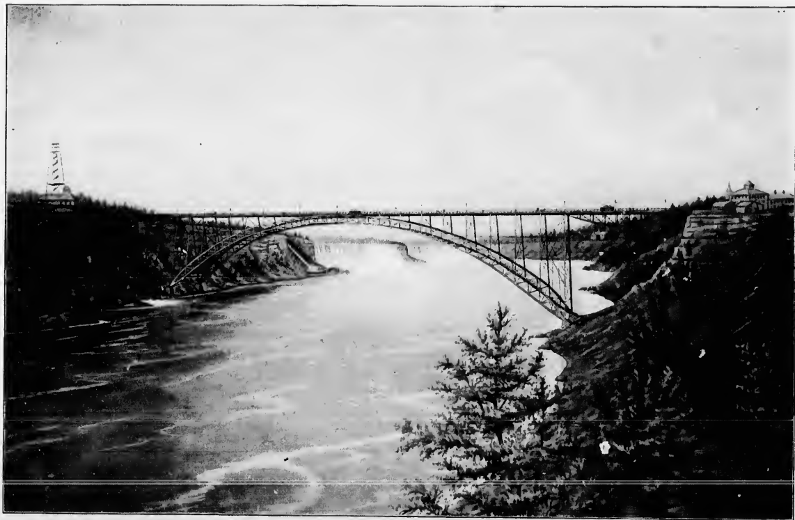
New Steel Arch Bridge, replacing Suspension Bridge.
