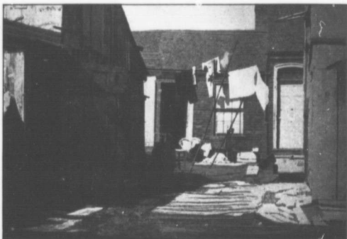
A corner of a courtyard in which over forty people dwell. Note the outside privies! Cut No. 13.
