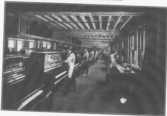
Action Placing, Regulating and First Tunings.
