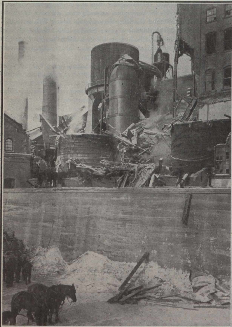
Wreckage from Sulphite Digester Explosion.
