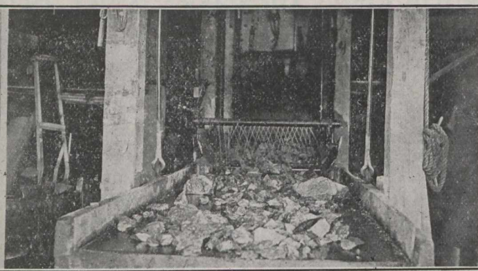
Bumping Table, Nipissing Jigging Plant
