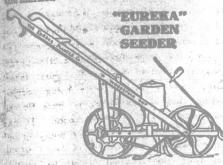
The only rear-wheel driven Seed Drill on the market. The Eureka will handle the most delicate seed without bruising or breaking and will sow evenly to the last seed. Can be instantly converted from a regular seed sower into a Hill-Dropper. No waste of seed when turning rows. For sowing Sugar Beets and all garden seeds this machine is unequalled. Sold with or without the Cultivator Attachments.
