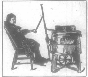
Ease in operation is one of the strong features of the "One Minute" Washer. The secret of this ease lies in the fly-wheel, under the tub, which runs on ball bearings. You push the handle one way and the fly-wheel forces it back to you.
