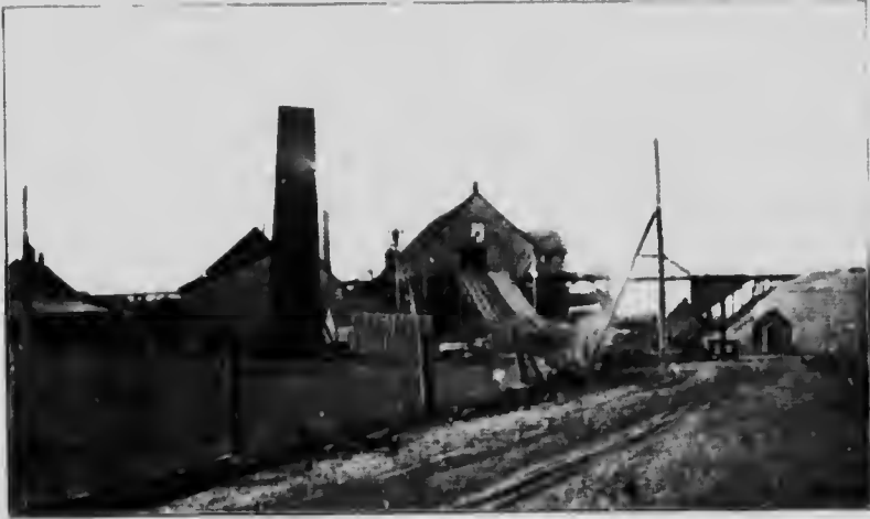
No. 1 slope of the Minnie Coal Company, River Hebert, N.S.
