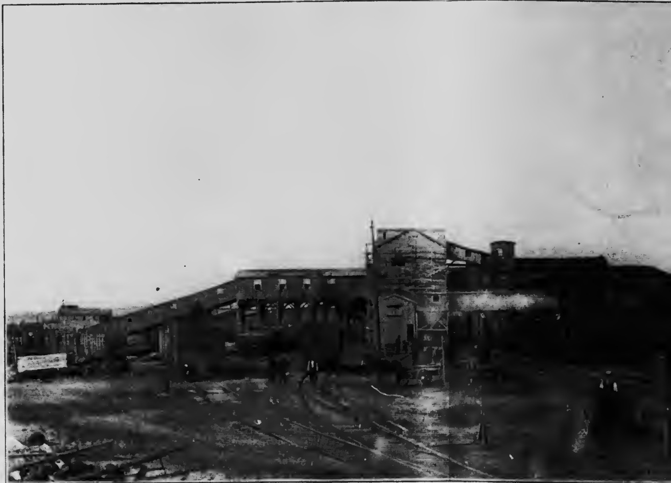
Bankhead and colliery buildings: Inverness Railway
