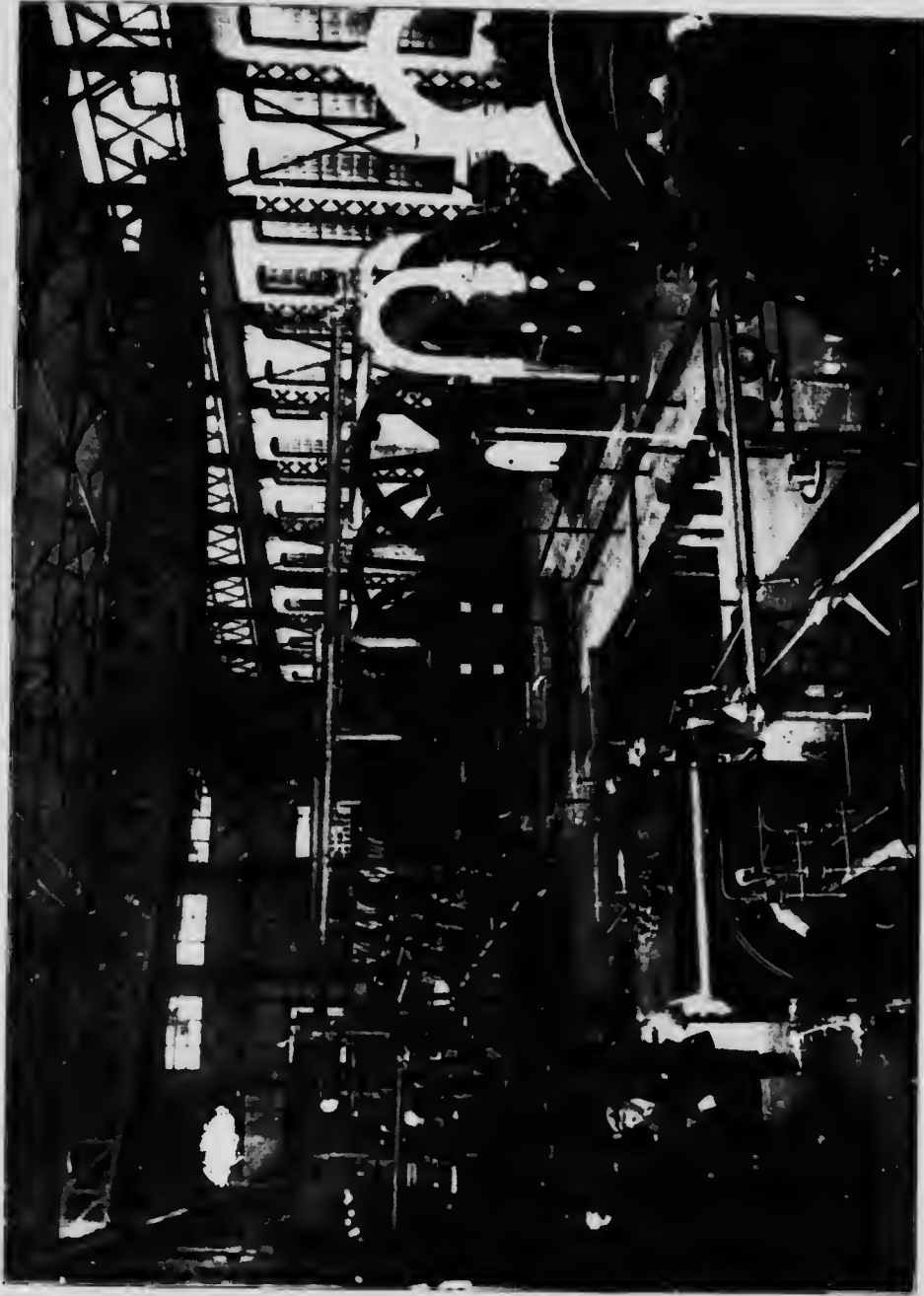
Interior of power house, No. 2 Colliery of the Dominion Coal Company, at Glace Bay, N.S.: showing air compressors and electric generators. The unoccupied space in the centre of the floor is now occupied by the turbo-generator set shown on Plate XXV.)
