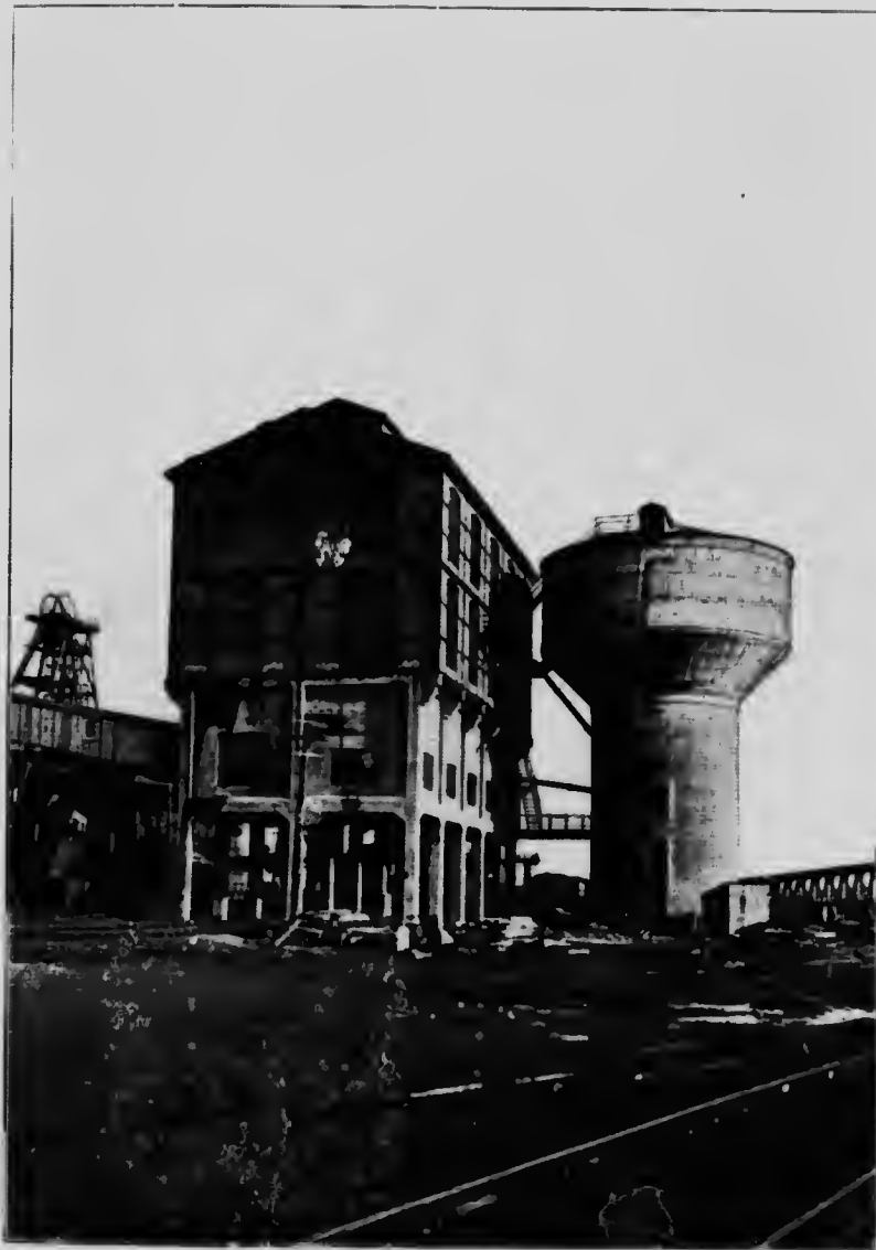
"Baum" coal washing plant of the Nova Scotia Steel and Coal Company, at Sydney Mines; showing washery and concrete settling tank.
