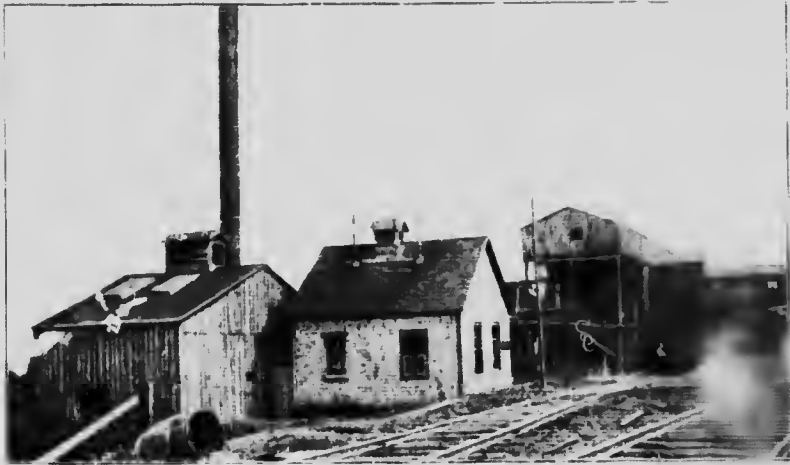
No. 2 slope of the Minnie Coal Company, River Hebert, N.S.
