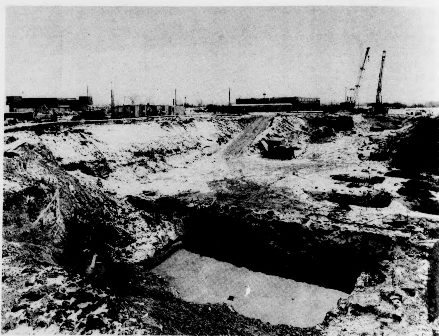
Mysterious pit that later became the beloved Ross Building.
